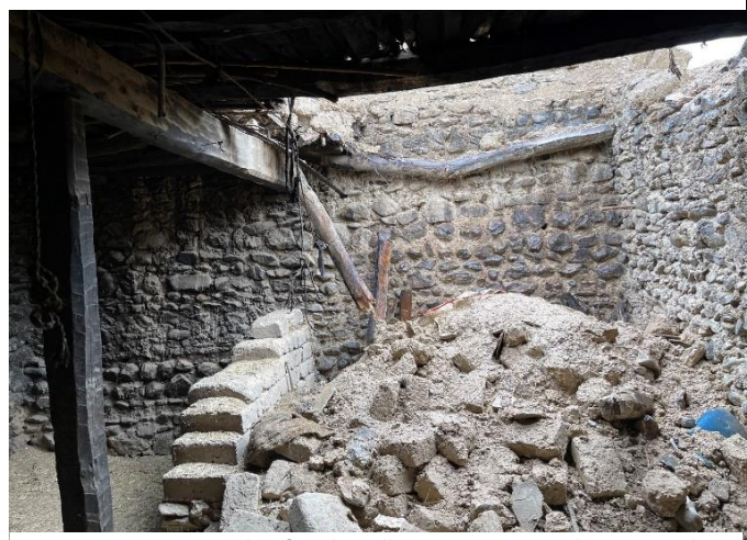
Figure 2-8. Example of rock wall construction to the rear with collapsed mud brick rubble in front.
