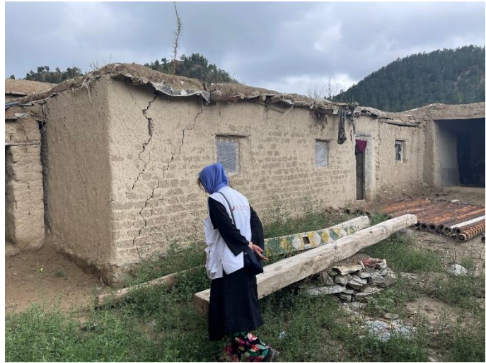
Figure 2-7 Example of mud brick construction.
