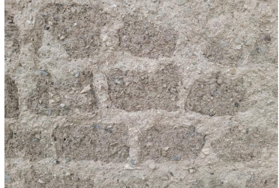
Figure 2-18. Example of plaster protecting mortar.
