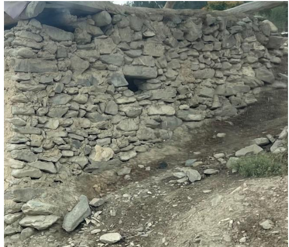
Figure 2-19. Example of angular rock wall construction.
