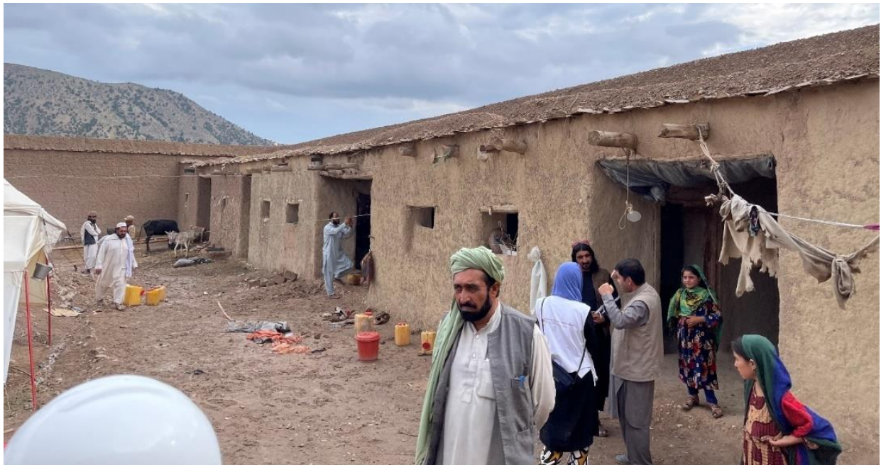
Figure 2-6. Example of Pakhsa used for inner compound room wall construction.
