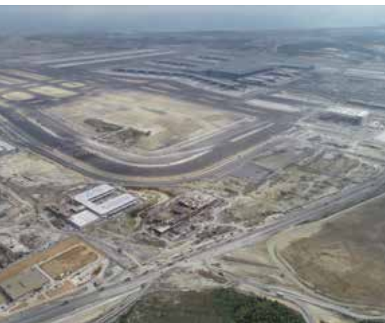
Turkey's new airport under construction in July 2018.
