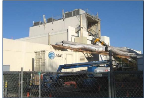
*Downtown Napa AT&T building was red tagged due to rooftop equipment anchorage failure and knock-out wall panel fallout.*
