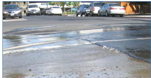
*Water bubbling up through downtown pavement - one of 120 water line breaks in Napa.*
