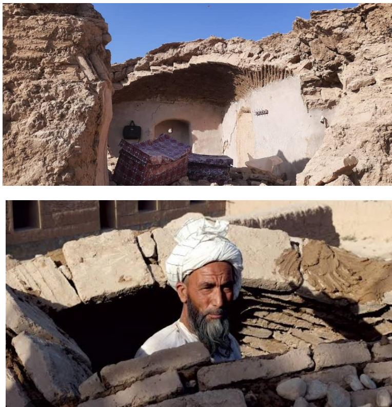
Figure 3 Domed roof construction process.
